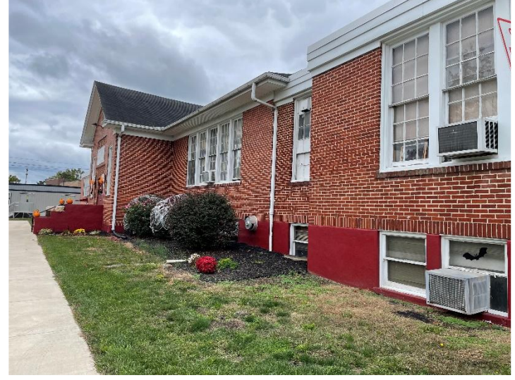
Current Inwood Primary to be demolished and new (PreK only) facility to be built on site.
