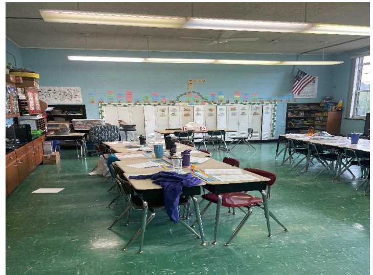
New HVAC, electrical and safe school entry will give staff and students a great learning environment.
