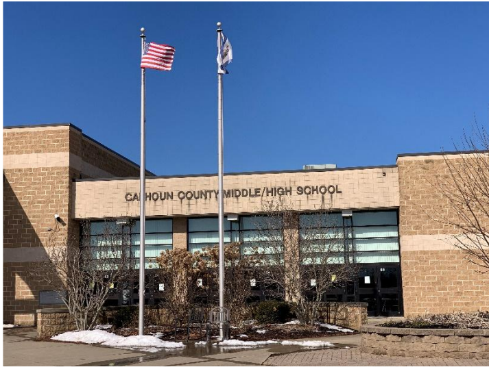
Calhoun County MS/HS was built in 1998 with SBA funds. Many systems are starting to fail due to their age.
