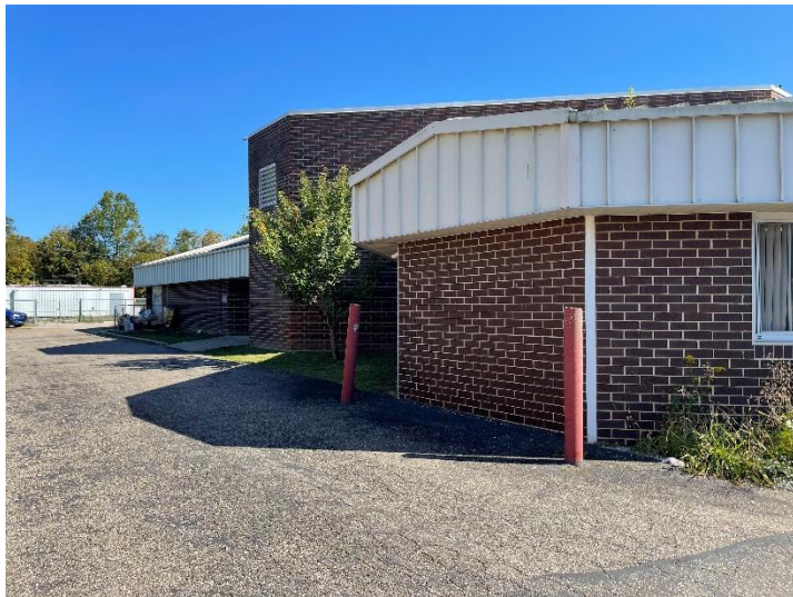
Location of the new two classroom addition.
