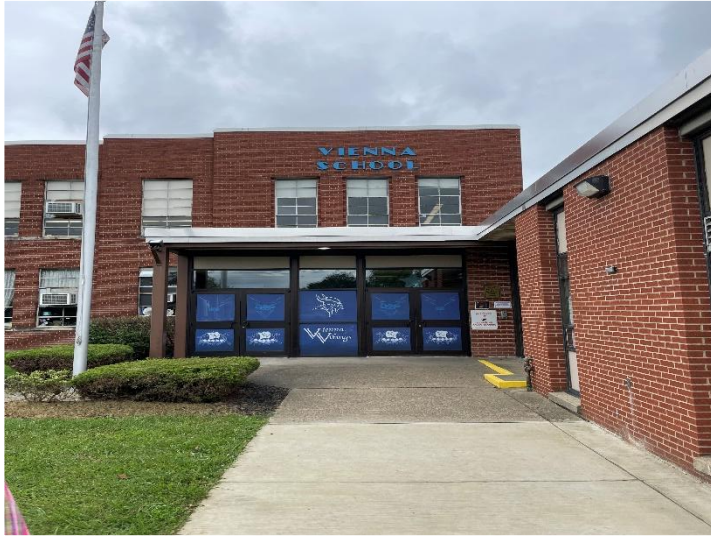
Wood County School's bond includes consolidated five existing elementary schools into three new schools.
